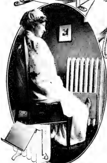
At left: A foot rest fastened to the radiator affords an excellent means of warming the feet
